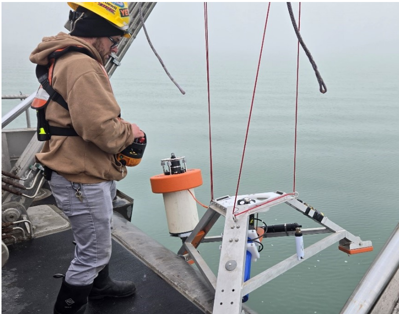
Figure 8. USGS R/V Muskie crew members lower an acoustic Doppler current profiler and other environmental data loggers housed within a tripod mooring near Niagara Reef in Lake Erie's west basin in December 2024.
